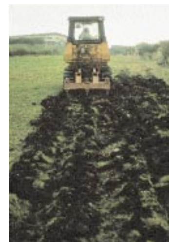
Ripping the site
