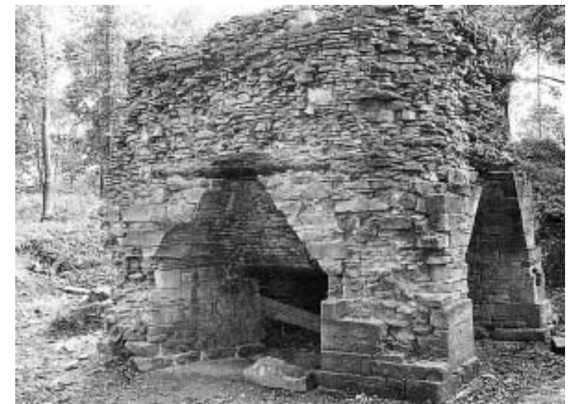
Rockley blast furnace was built around 1700 and was fuelled by charcoal throughout the first half of the 18th century
