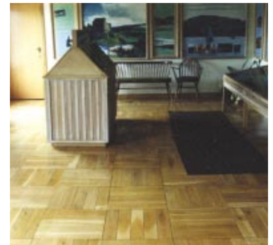
End grain floor tiles made from small roundwood timbers are extremely hardwearing and very attractive
