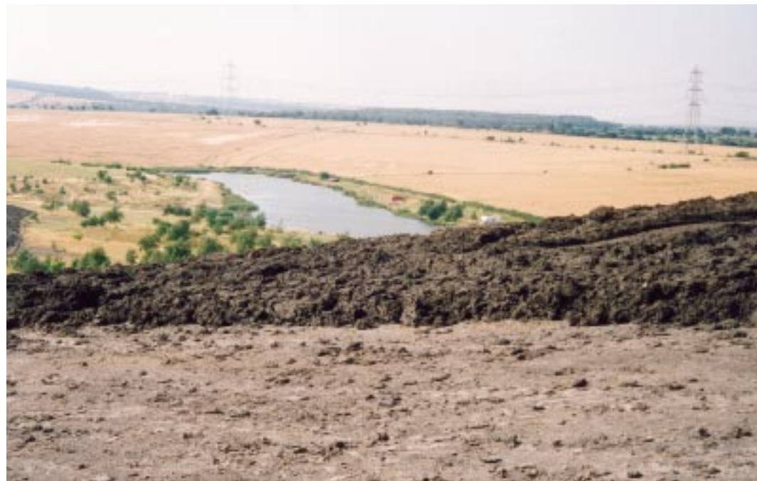
100mm of biosolids spread ready for incorporating into waste-tip surface
