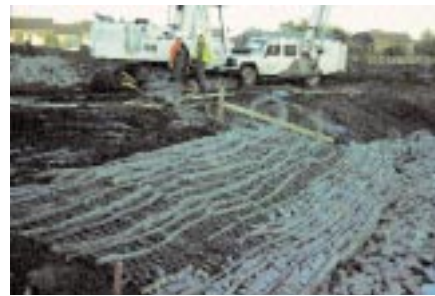
Willow matting under construction
