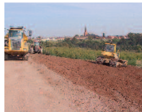
Figure 1 Appropriate use of soil materials is essential in any reclamation project.
