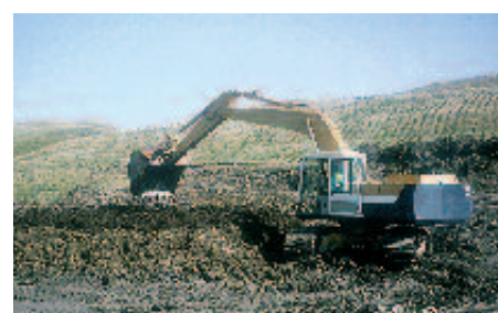
Figure 1 Reinstatement of soil materials using the loose tipping method.
