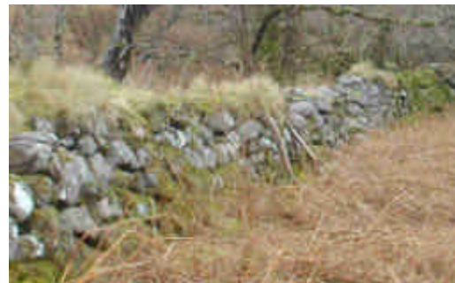
r: Woodland enclosure dyke, Glen Liver
