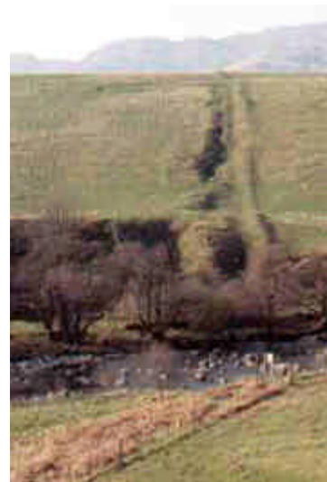
r: massive earth dyke at Glenartney
