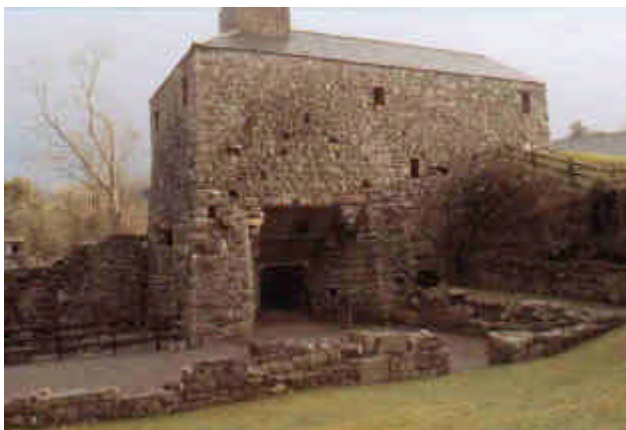
Bonawe furnace, Loch Etive
